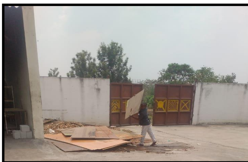
Separate place for Construction wastes at ACE, Hosur, Tamilnadu.
