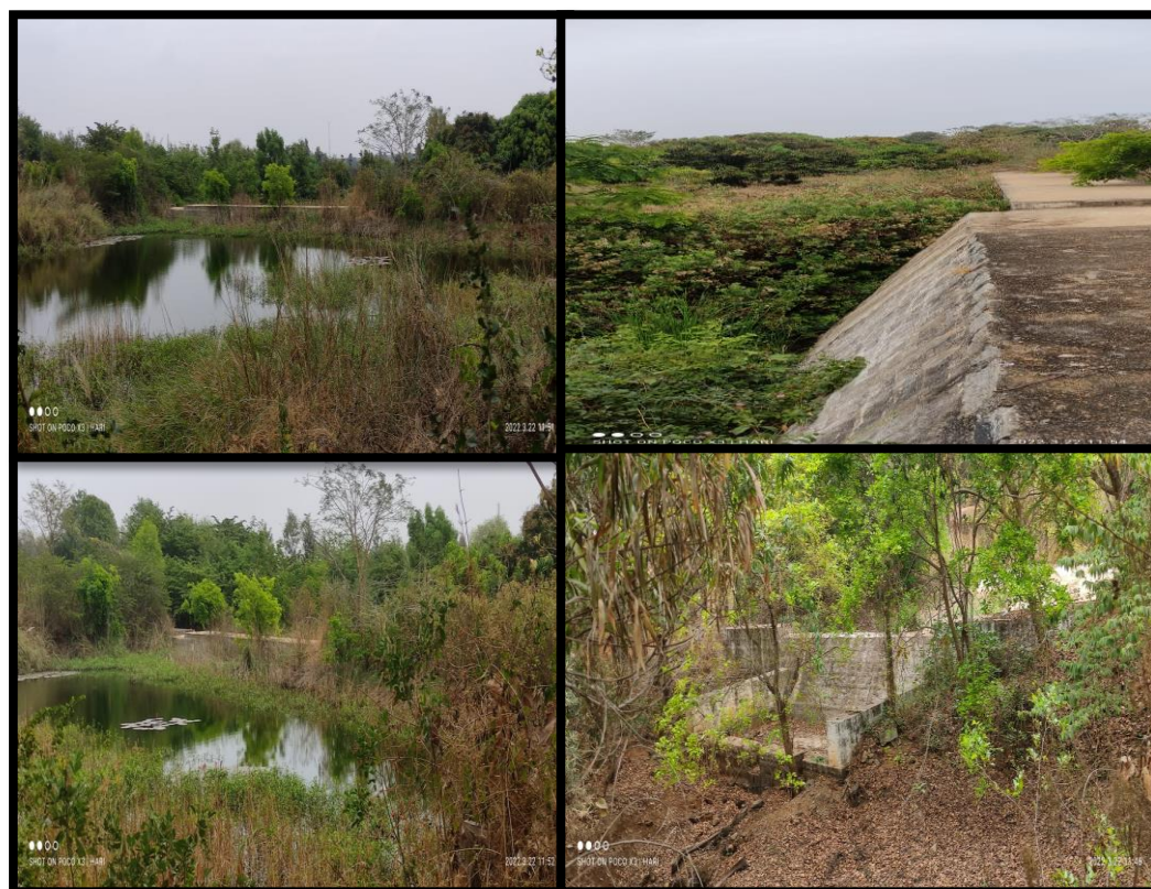
Construction of check dams in ACE, Hosur, Tamilnadu.
