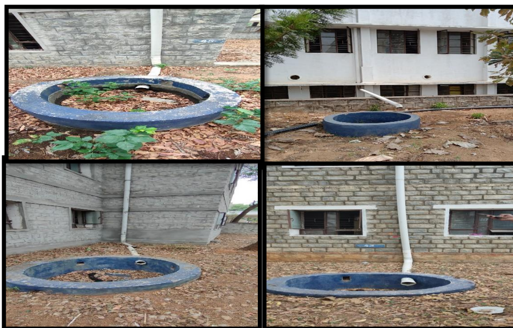
Rainwater harvesting units in ACE, Hosur, Tamilnadu.
