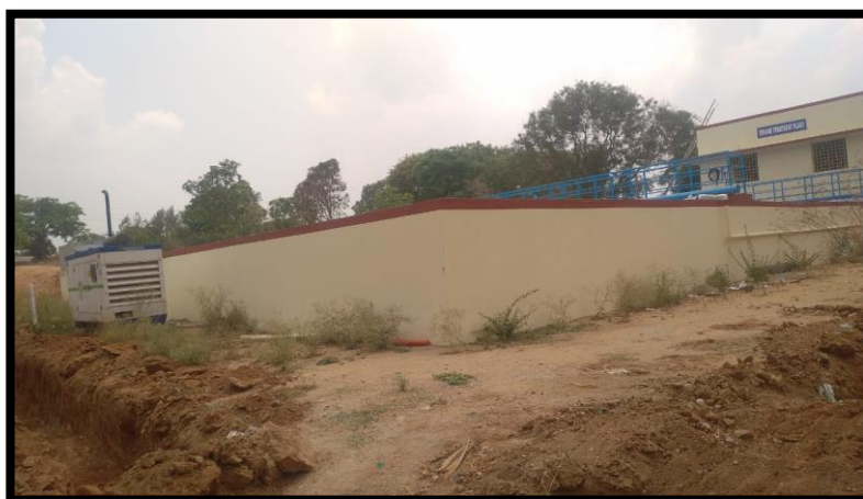
Sewage Treatment Unit in ACE, Hosur, Tamilnadu.
