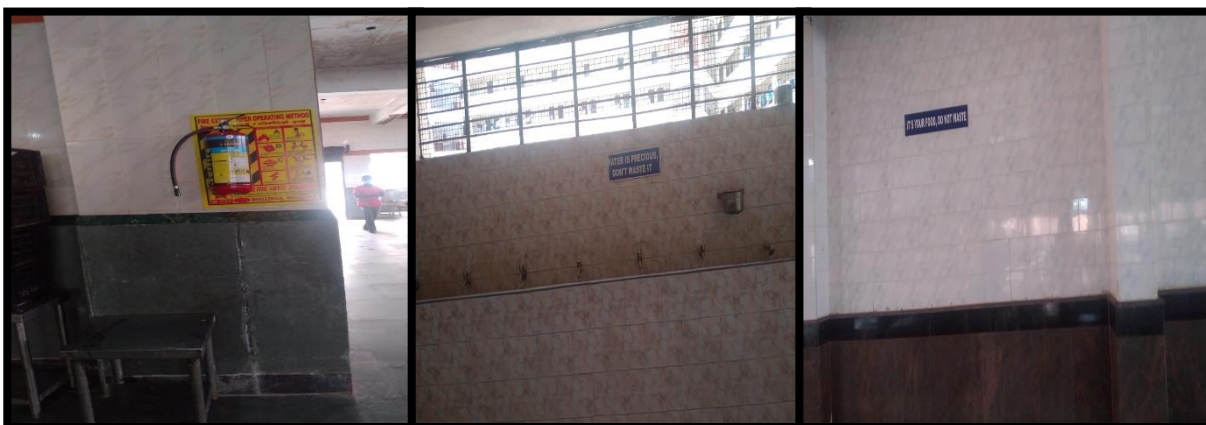
Safety measures at ACE, Hosur, Tamilnadu.
